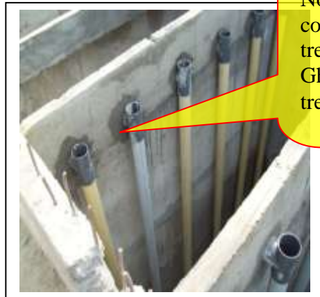
Baffled Reactor under Construction
