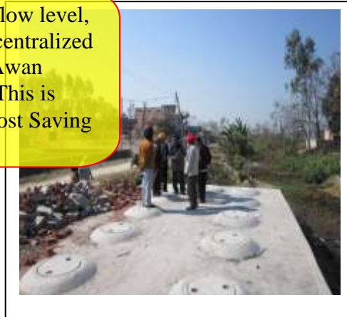
Baffled Reactor Complete
